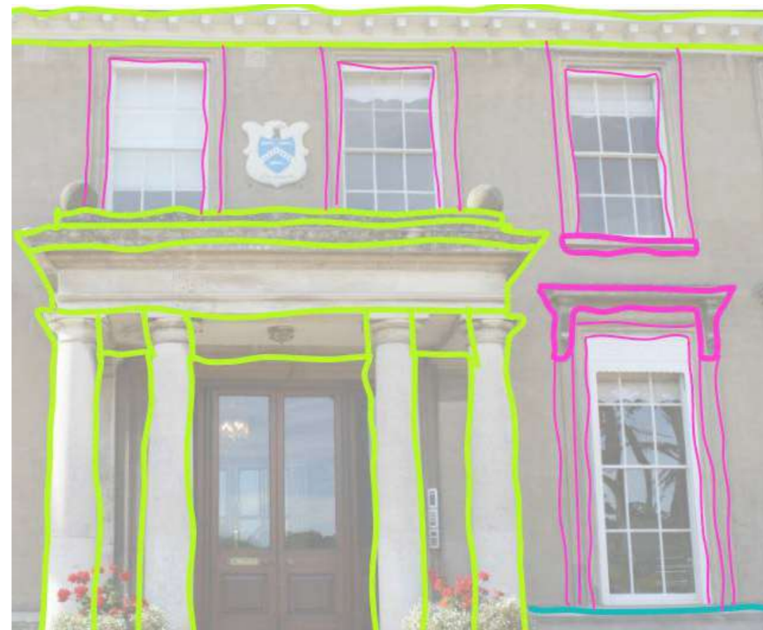
Douces Manor: Georgian order of façade, stacked openings, detail added through depth
