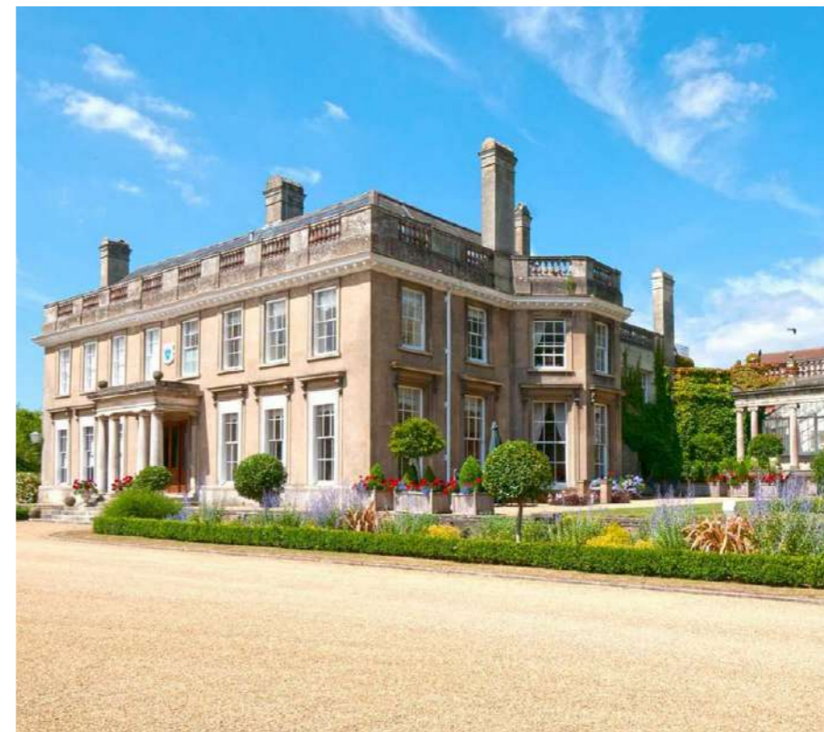
Entry Clearing: Building reveal from formal entry sequence
