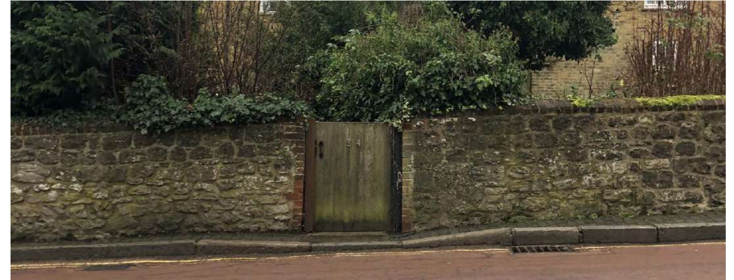
Typical landscape features: Ragstone and brick boundary wall leading to monastery grounds
