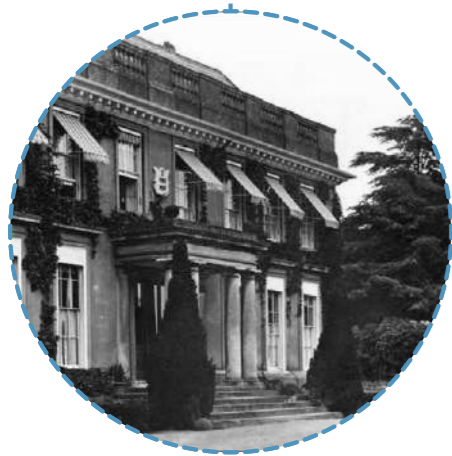
Historic image: Integration of building and landscape and window shading awning features
