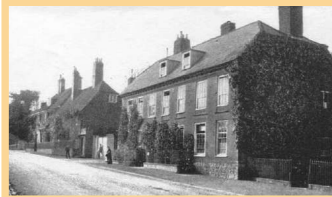
Sub Area A - Historic and Commercial Core High street typologies, order of façades and materials
