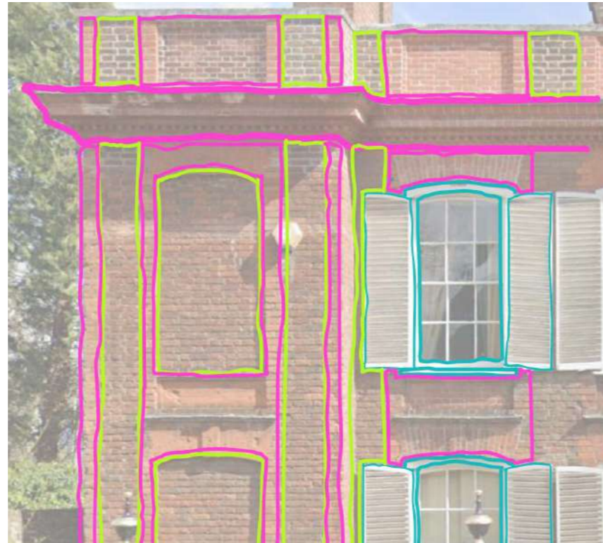
Went House: Georgian order, stacked openings, brick articulation, window shutter detailing
