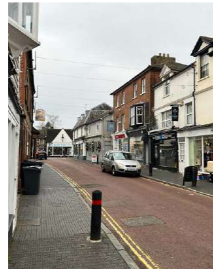
Swan Street looking West: Narrow street with variation of two storey pitches, mix of brick and render with shop frontages
