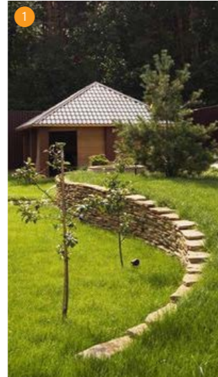
Kent Ragstone low retaining walls
